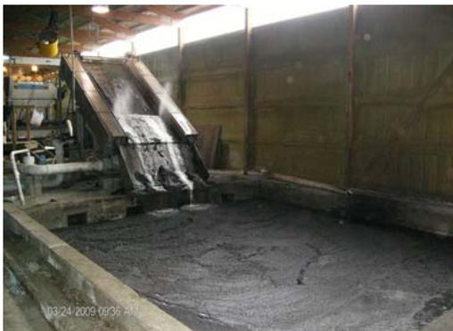
Suspended solids are removed using a microscreen separator and polymer
