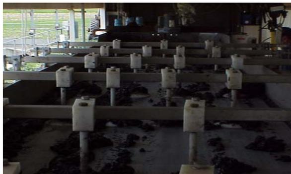
Suspended solids are separated using a gravity belt thickener and chemical flocculent
